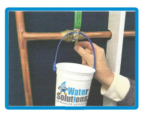
2. Most shut off's have a drain cap underneath. After you have turned the shut off to the "off" position, place a bucket underneath and open the small drain cap to allow water to drain back.
