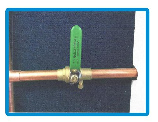
1. Shut your water to the sprinkler system off. The shut off valve is usually located in your basement.
