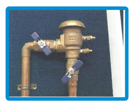
3. After steps 1 and 2, go outside to your pressure vacuum breaker (PVB, Backflow) and turn the handles to a 45 degree angle as shown in the picture below. You can also turn the screw slots on the test cocks 45 degrees. Once you open the test cocks it will start draining water back into the bucket inside.
