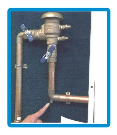
4. Most backflows have a drain elbow under them. Remove the cap and make sure the gasket comes with it. Put the cap in a safe place where you can find it in the spring.
